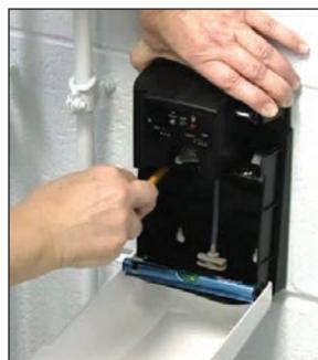
2. Open the dispenser and hold it flat against the wall. Using a pencil and the screw holes in the back panel of the unit, mark where to drill the screw holes. Using a M5 (5 mm) drill bit, drill the holes.
